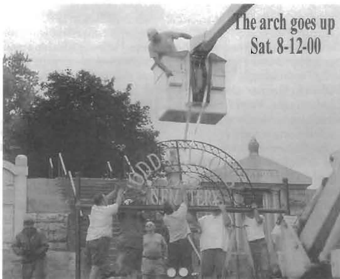
Shouting advice such as "Easy does it!" and "Careful!", one dozen workers manipulate a 550-pound steel arch and secure it to a cross beam at Tamaqua's Odd Fellows Cemetery pedestrian entrance. The ornate arch replaces a similar one; an early community landmark sacrificed about 1941 to help the war effort.
