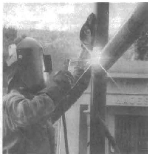
An early morning glow in Tamaqua wasn't only from the peeking sun, but from a welder's torch. John Schickram, Hometown, welds steel supports in preparation for the historic return of Odd Fellows arch, gone from the scene for close to 60 years.
